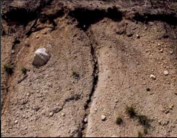
Erosion – Surface erosion.
