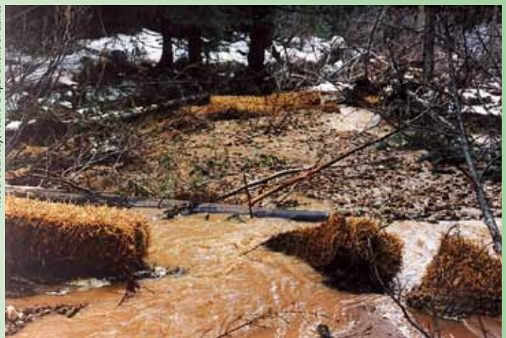
Failed straw bale check dam.
