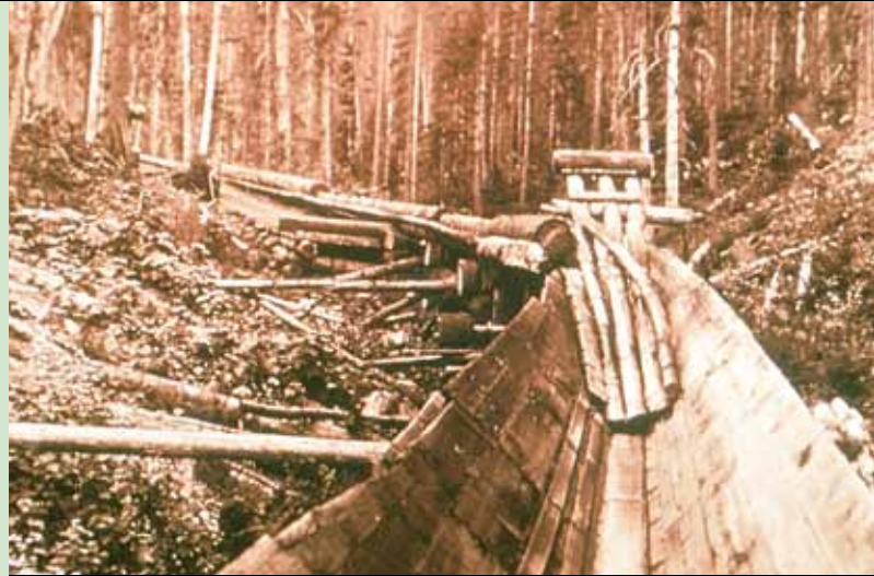
Logs being moved downhill in a flume.
