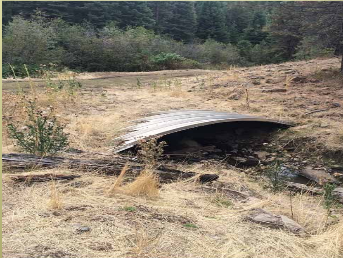
Culvert replaced with large arch for fish passage on Eight Mile Creek.
