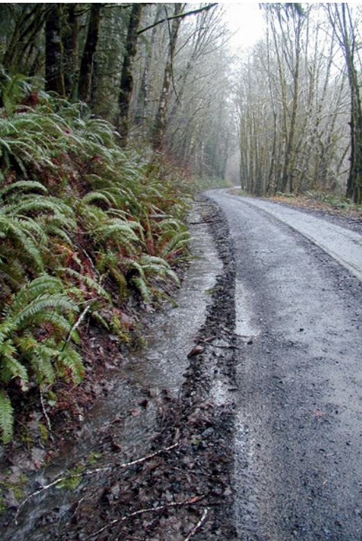
Durable rock surface on a log-hauling road during heavy rain. Notice that the water in the ditch is clean.
