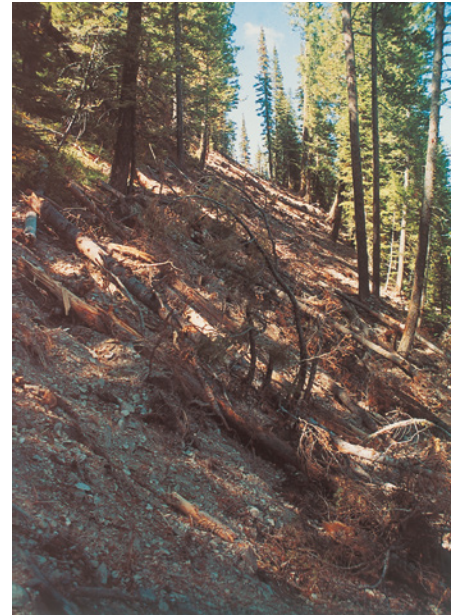
Vacated road segment with large wood in place, before reseeding the surface with grass.
