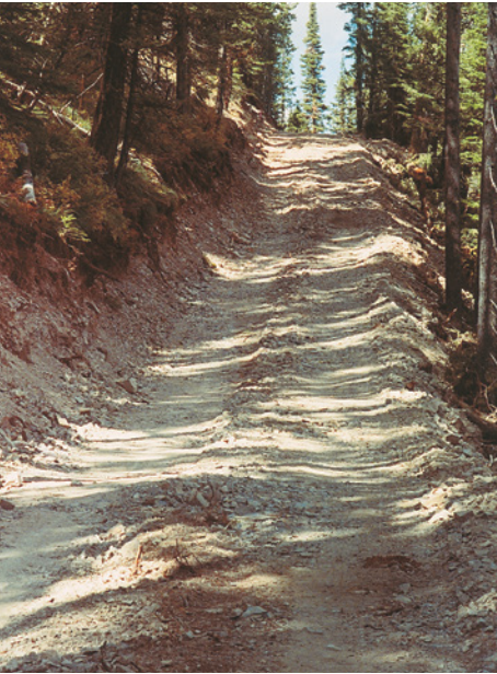
Road segment before vacating.
