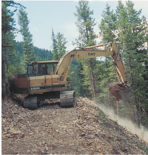
Excavator dismantling the road corridor.
